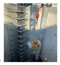
Handling of segments for placement in a tunnel constructed using a tunnel boring machine.  $\rightarrow$
